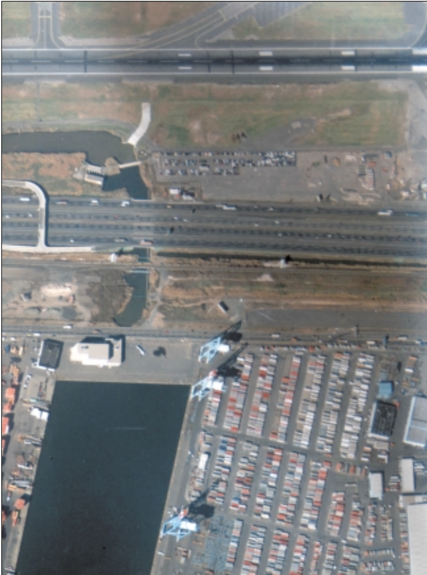
Photo 1. An aerial view shows some of the affected area. One part of the project involves relocating the railway line with a fly-over to cross above McLester Street. Currently, the railway line crosses the main north-south roadway, Corbin Street, at the same grade level, causing traffic delays numerous times each day as trains travel through the intersection.
